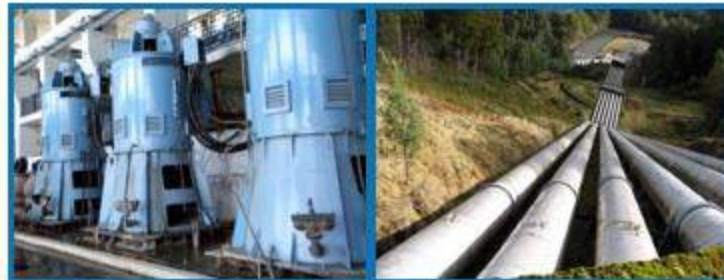
Water Pumping & Distribution
