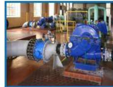
Waste Water Pumping
